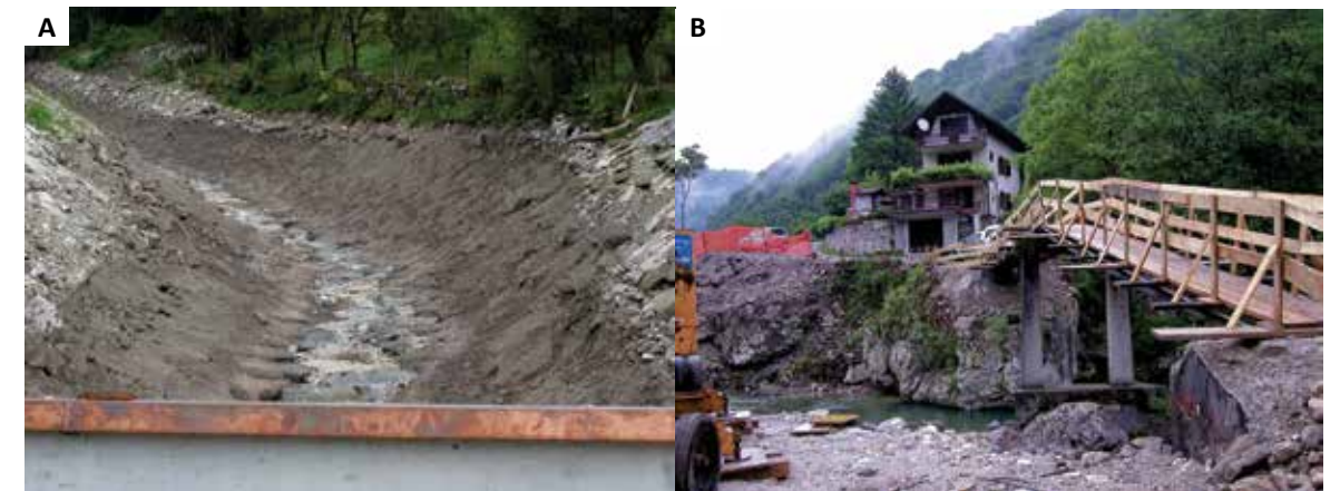
Fig. 25: Mitigation measures. A- Enlarged parabolic channel cross-section of largely constant longitudinal slope and no sharp curves; B- Implementation of a new bridge with nearly twice the span of the old bridge to connect the two parts of the village.
