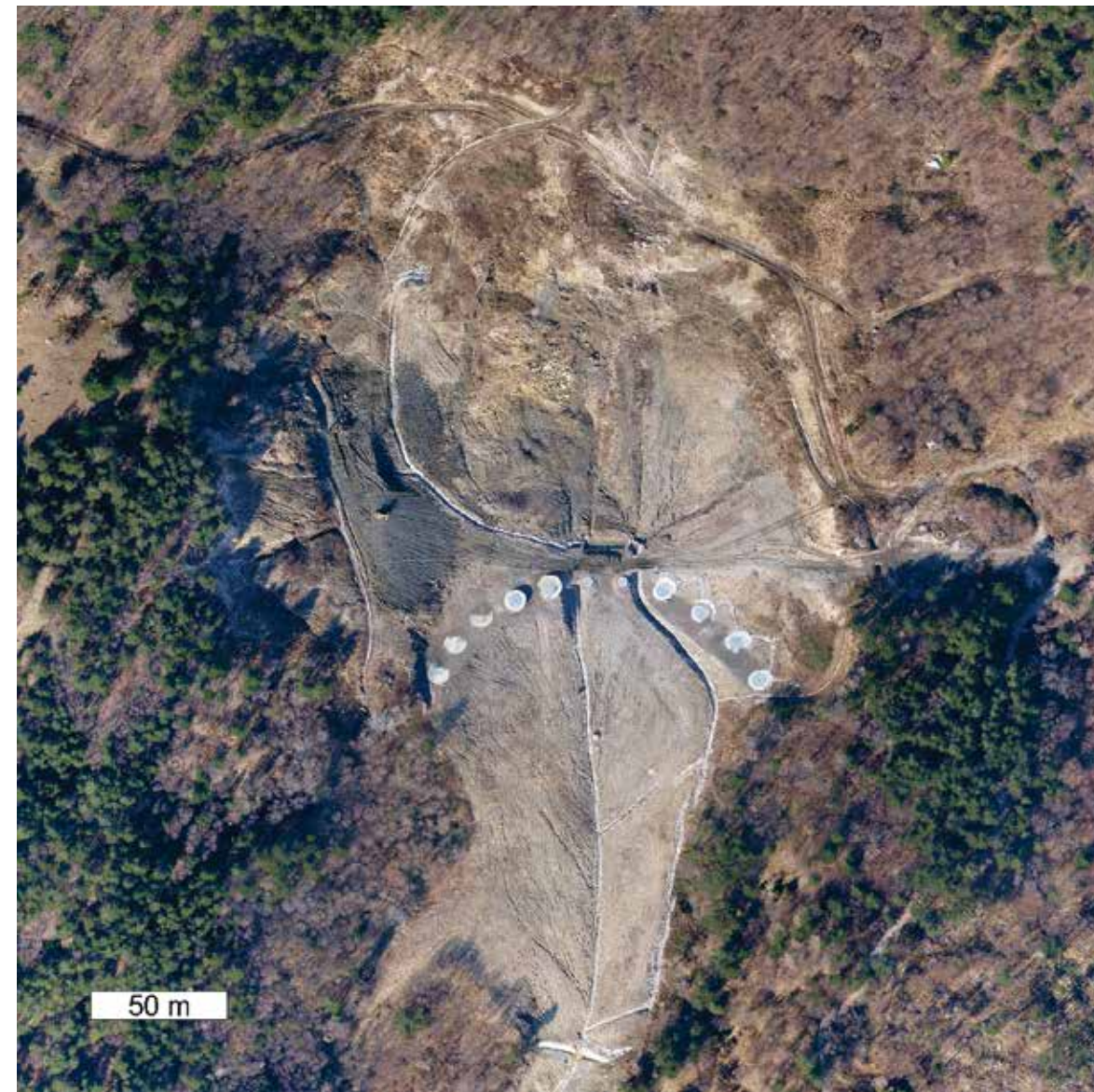
Fig. 16: Aerial view of the upper part of the Slano blato landslide with shafts and a small concrete dam (Pulko et al., 2014).
