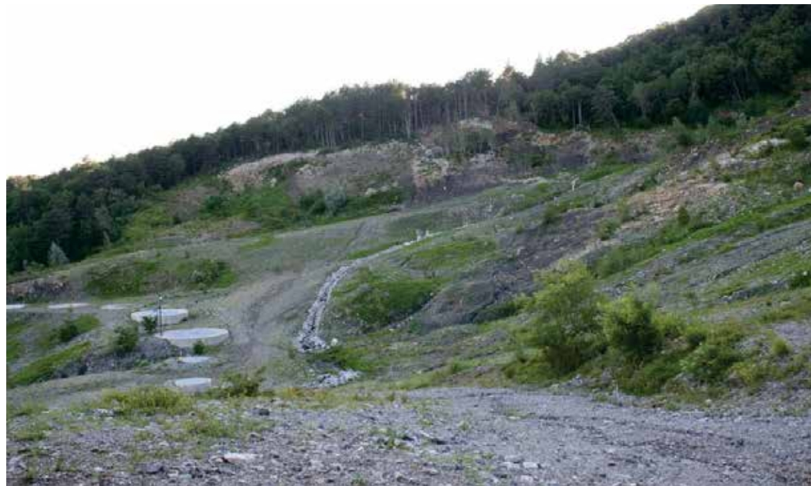
Fig. 18: Upper part of the Slano blato landslide above shafts in 2011.
